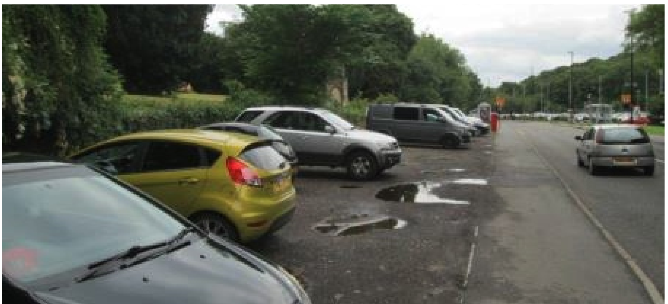
Unsuitable frontage to the Listed Licensed Victualler's Almshouses
